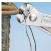
Quick and comfortable twisting and cutting of binding wire
